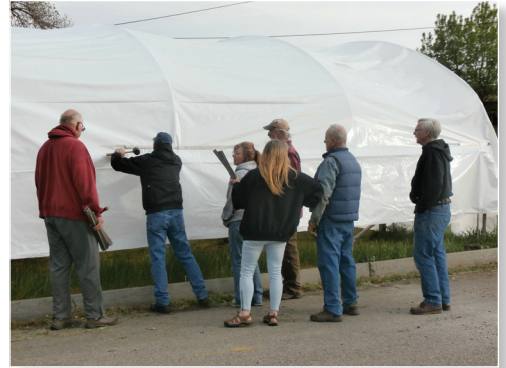
2015 Greenhouse Cover Installation
