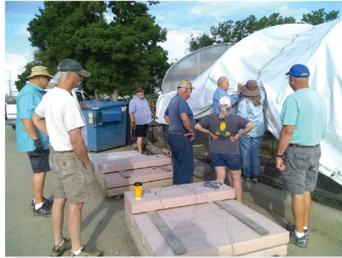
2020 Greenhouse Cover Installation
